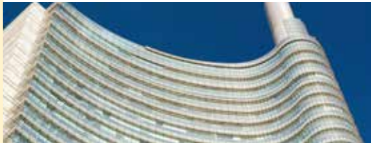
Offices and business centres
